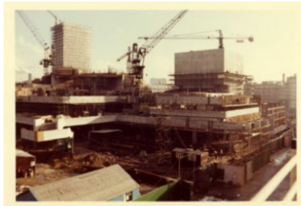
The National Theatre building took seven years to complete. Image: Courtesy of Sir Robert M c Alpine
